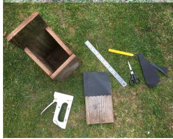
6. Measure out and attach a piece of rubber to use as a hinge for the roof. The rubber hinge will allow you inside to clean out the nest box in winter and will provide a bit of waterproofing for the top of the nest box. Used a staple gun and staples/ hammer and nails to attach the rubber hinge.
