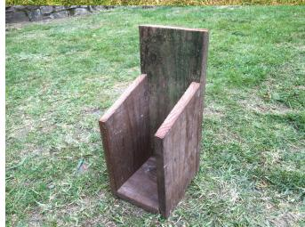
5. Assemble the pieces of the nest box minus the roof. The back board, sides and front wrap around the base piece. If you are using a drill, pilot holes using a drill piece slightly smaller than the screws can help make it easier to assemble. Ensure hair is tied up and out of the way for drill use! Attach the side pieces to the backboard first, then the base and finally the front.
